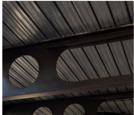
2. Base Build beams and soffit
