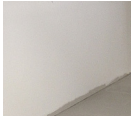
3. Base Build Plasterboard
