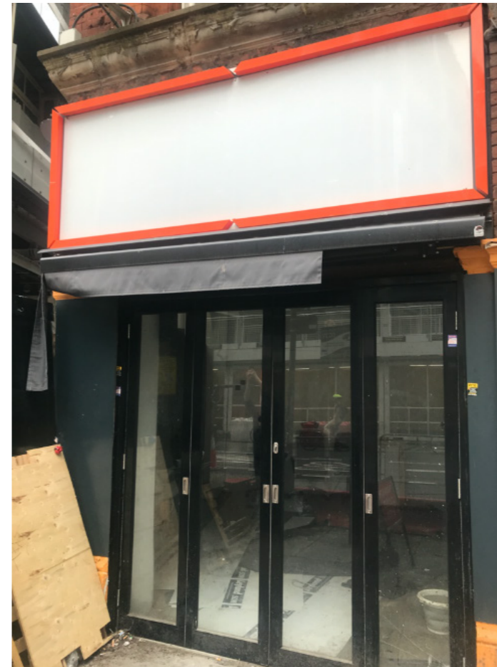
Figure 1 Front Elevation of the Vacant Unit
